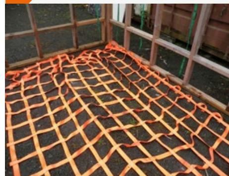
**Inspect the net** for any damage prior to install, record this in your visual inspection register with serial number, date, time and sign off.
