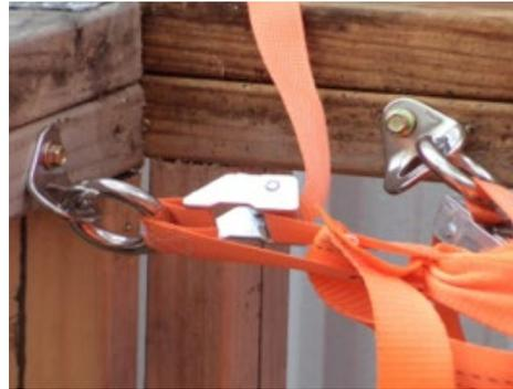
Use the hangers if you have gable ends or larger lintels. Use a type 17 14 gauge 75mm screw & screw hanger to the top plate, (*Screws can be used only once*) **place hangers at 450mm centres maximum spacing.**
