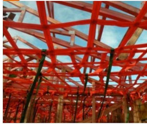
**Where joining of nets is required** overlap webbing of nets 3 full squares and secure with cam buckle straps on every second square on alternating sides.
