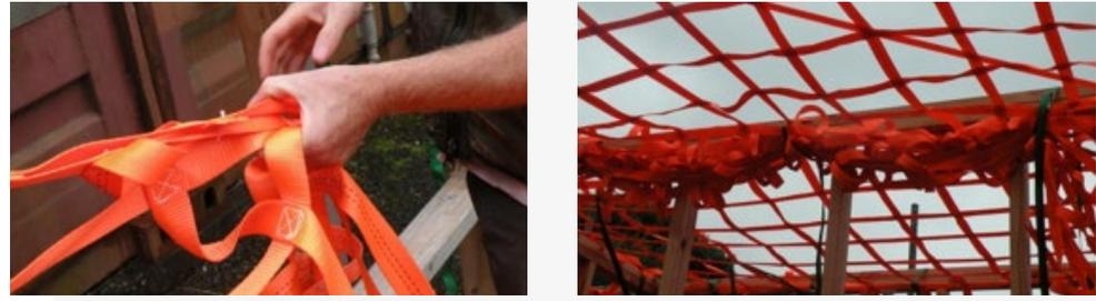
**The net should have some sag, 100mm minimum and 400mm Maximum.** There should always be a minimum clearance under the net of 2 meters to allow clearance for the net to absorb a fall.
