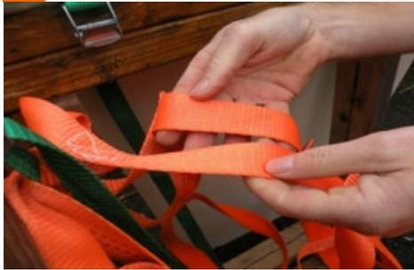
Starting in the corner of the room wrap cam buckle straps (*use only Stop Drop branded straps*) around double top plates **and through 2 webbing strands**.
